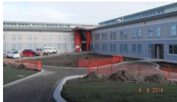
Construction in progress at Wiri. Photograph courtesy of SecureFuture.
